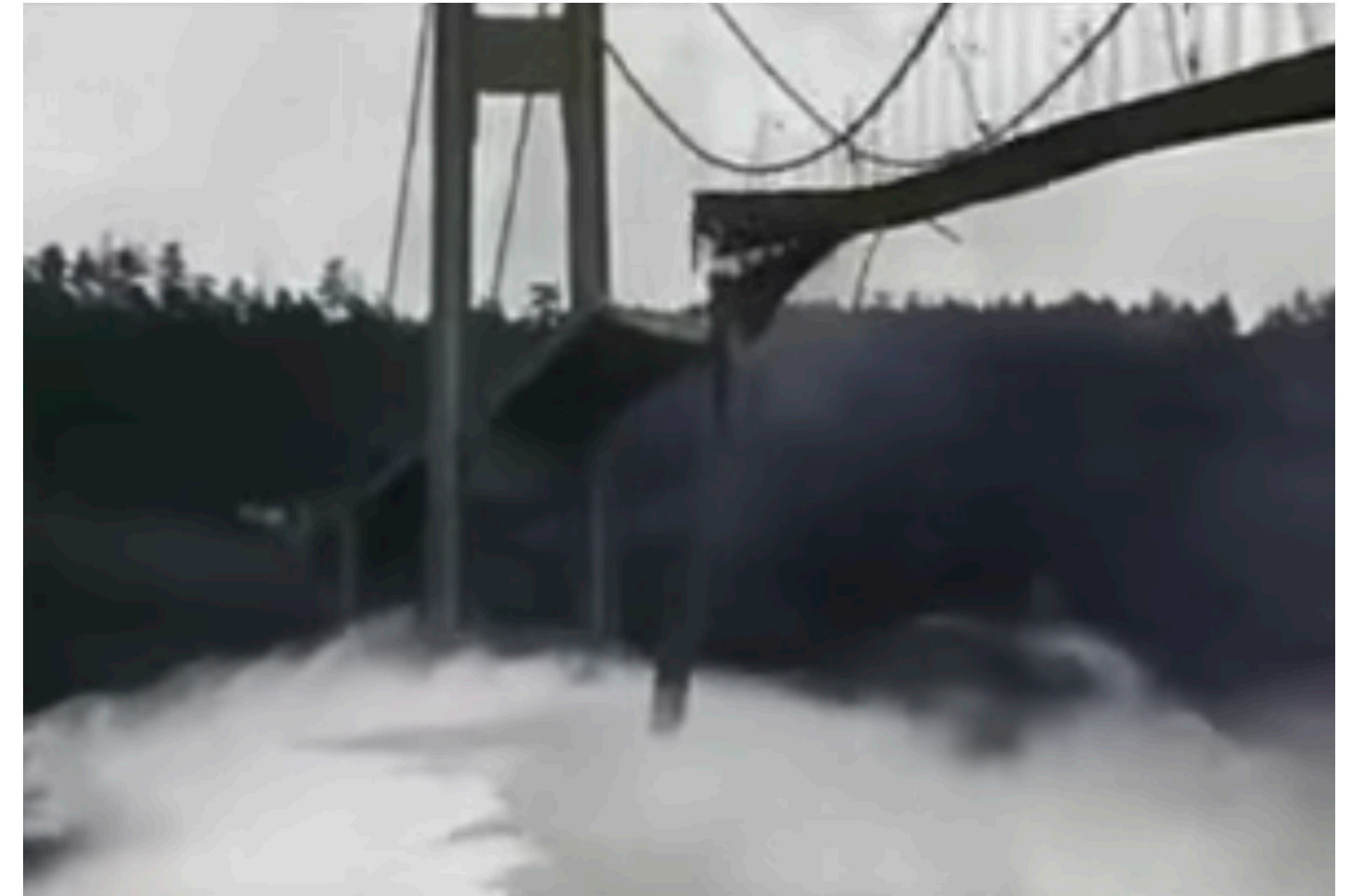
Tacoma Narrows Bridge
